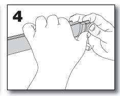
When all brackets are in place, clip the stop-end to the gutter. Some force is necessary in order to compress the rubber seal. A smear of washing up liquid or silicone grease/spray on the seal may help if required.
